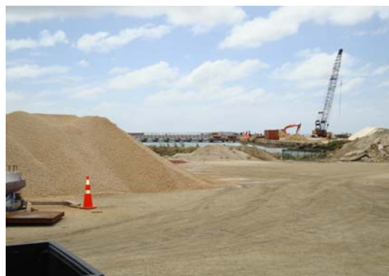
Construction of Vuna Wharf
