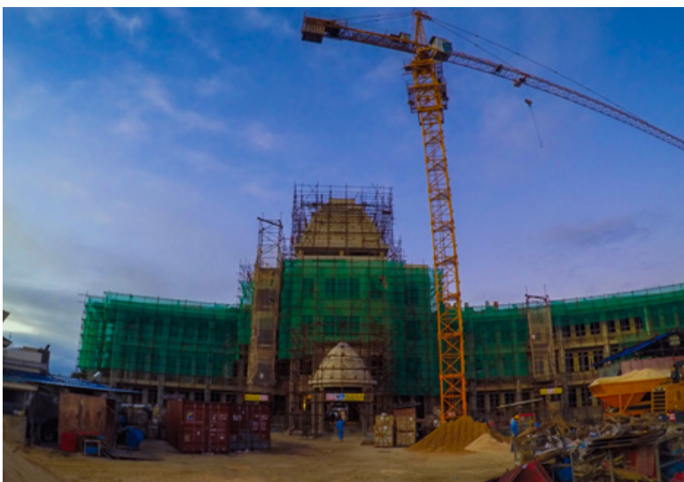
Construction of the St. George Palace, Nuku'alofa, Tonga.
